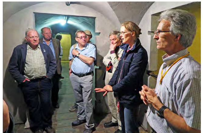
Central space in the cruciform of Mussolini's final unfinished bunker. Each cross chamber should have had blast doors but these were never installed
